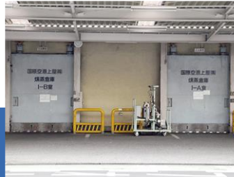
Fumigation Facility : 466㎡ Function : Exterminate/sterilize disease and pest from agricultural products
