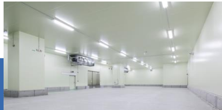
Temperature controlled room (-20°C) : 435㎡ Main Cargo : Frozen foods,Pharmaceuticals,etc
