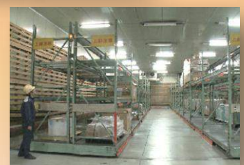
The door and inside of the +5°C refrigerator at A-Wing.
